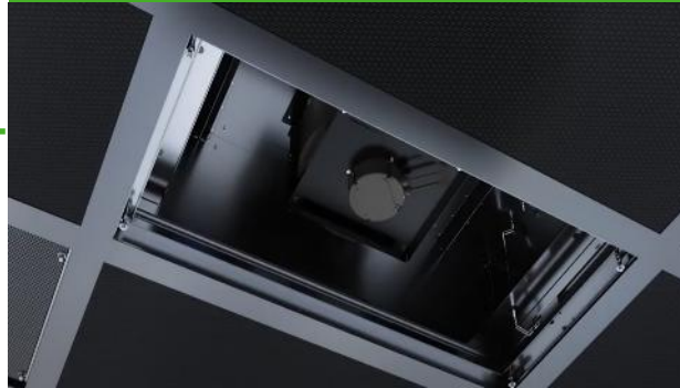
2. Cleanroom ceiling from below
